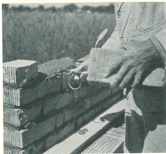
Bindaren muras in i yttre 1/2-stensmuren
